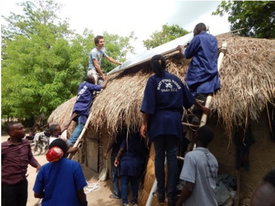
Installation of the prototype (May 2018)
